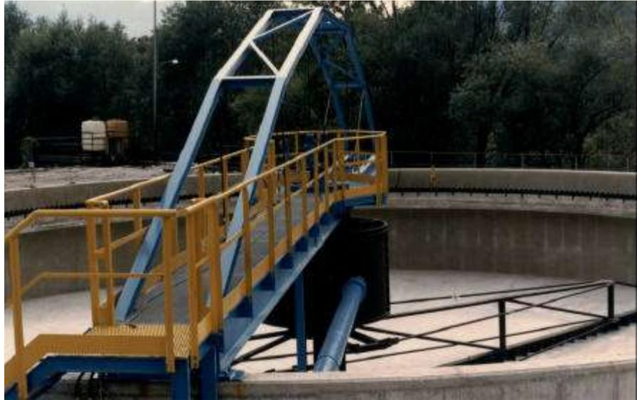
*The scraper support arms are connected to the vertical shaft and manufactured with suitable bracing from rolled steel sections, to form a rugged construction preventing deflection or distortion when operating under load conditions.*
