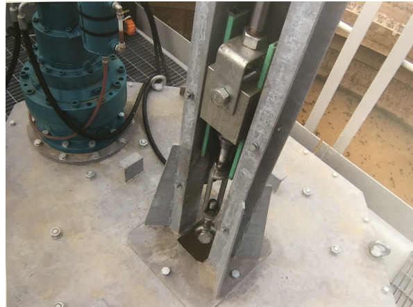
Hydraulic scraper lifting system – Detail without safety protection
