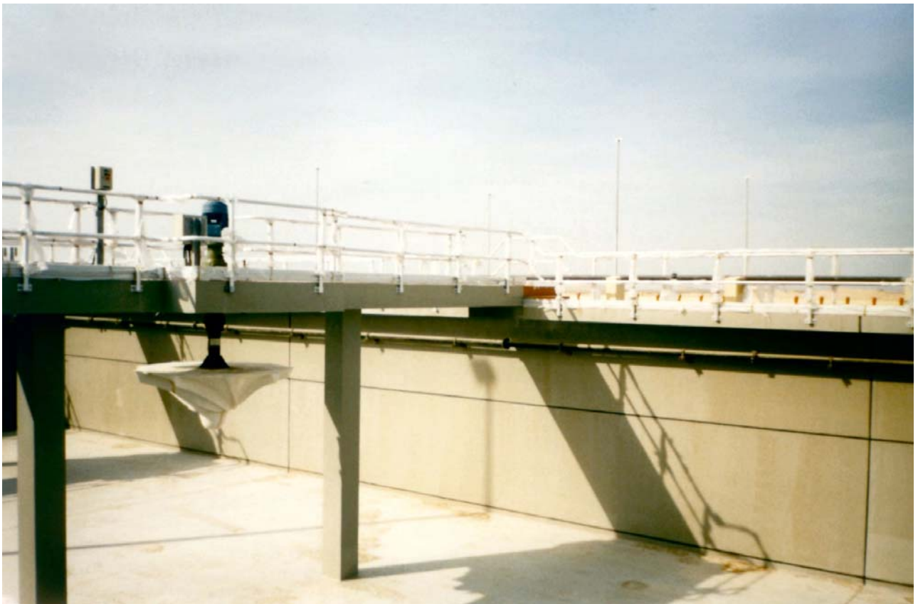
Impeller dia. 2700 under construction
